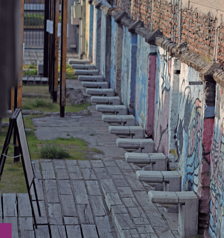
Muro interior Interior wall
